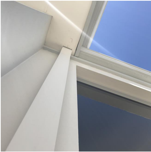
4.1.1b. Roof External fascia movement
