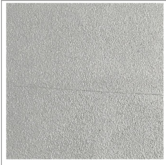
4.2.1d. Minor cracking
