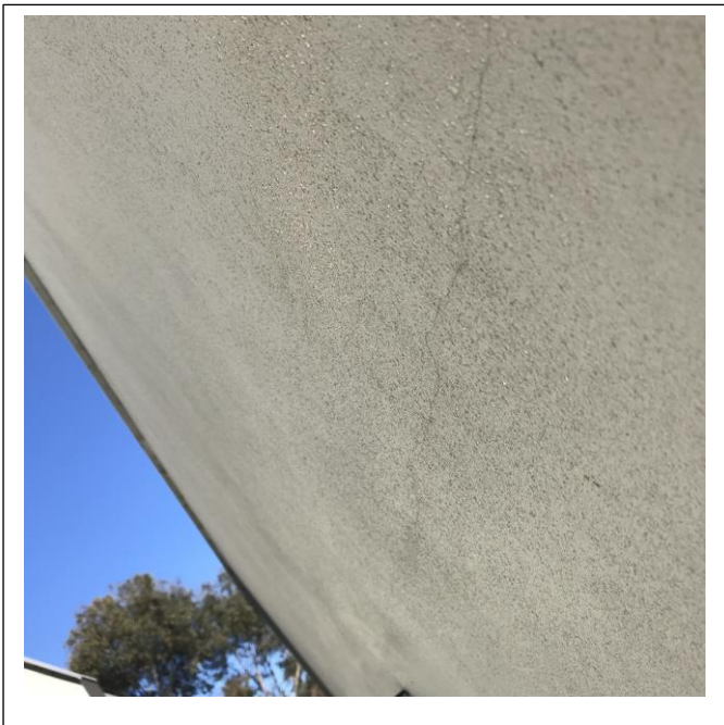
4.2.1d. Minor cracking
