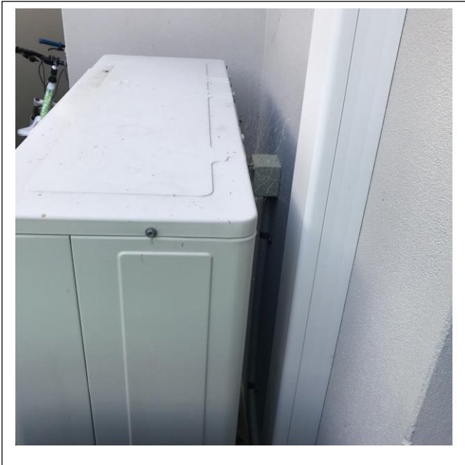
4.23.1a.No chains on air conditioning units
